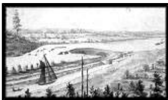
Hog's Back Dam & Locks c 1840
